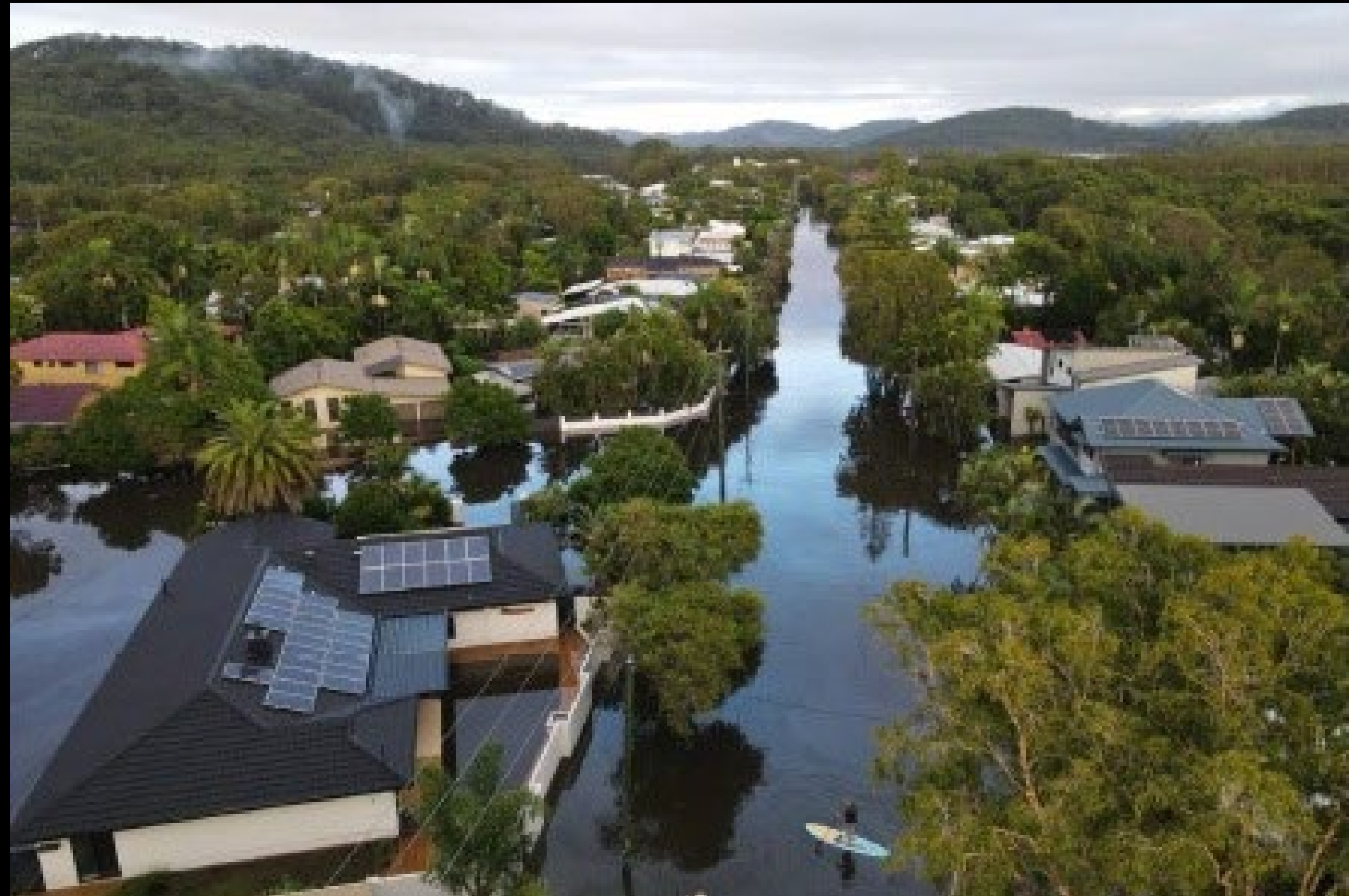
Cabarita & Bogangar flooding, April 2020
